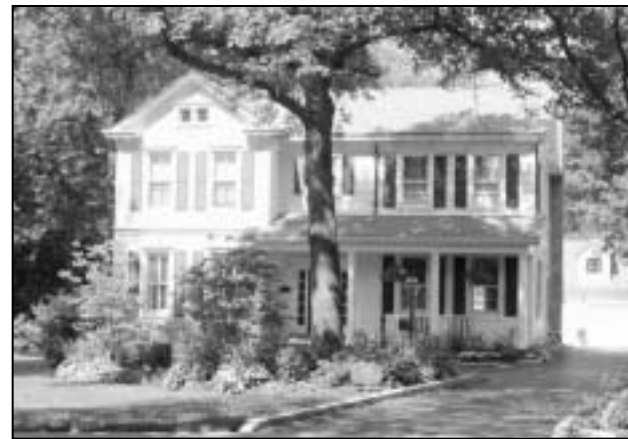
No. 60 Kinsella House 745 North Taylor Avenue, c. 1872
