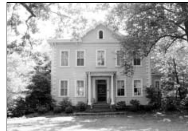
No. 31 Keith-Greensfelder House 116 North Woodlawn Avenue, 1850
