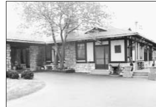
No. 45 Lemp Estate: "Cragwold" Built 1911
