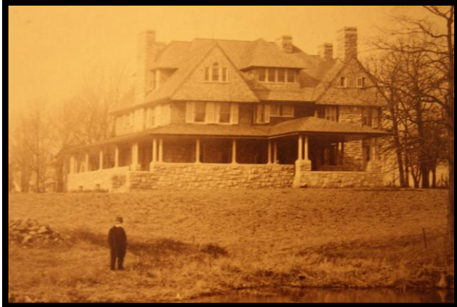
Demolition of Landmark Landmark #79, Brownhurst, c. 1892
