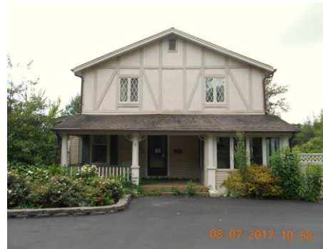
632 EAST JEFFERSON AVENUE
