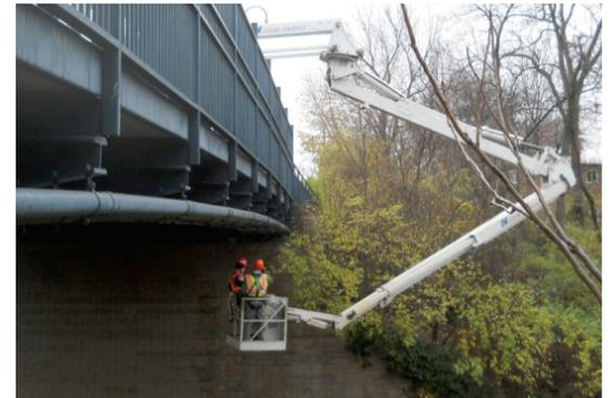
**SNOOPING AROUND:** Engineers from Horner and Shifrin were transported via their "Snooper" truck to inspect the underside of the Clay Avenue overpass recently. Photo by Kirkwood Street Department Supervisor Doug Thrasher.
